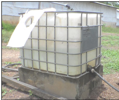
Figure 3: a tank, power supply
